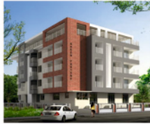
Green Fortune End point, Manipal
